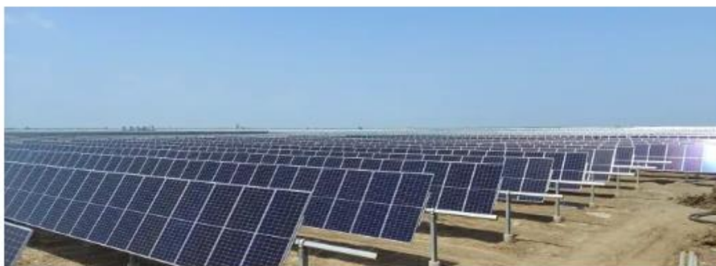
300MW Single Axis Tracked at Dholera
