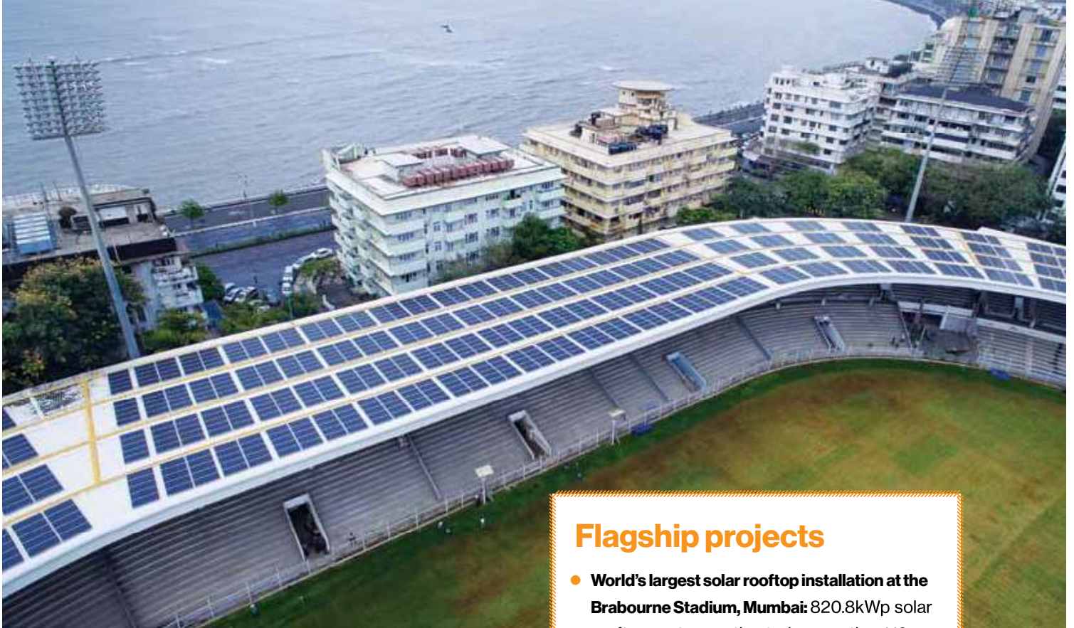
Solar rooftop panels installed at the Brabourne Stadium, Mumbai
