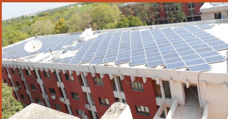
Hartek Solar’s rooftop project in Chandigarh
