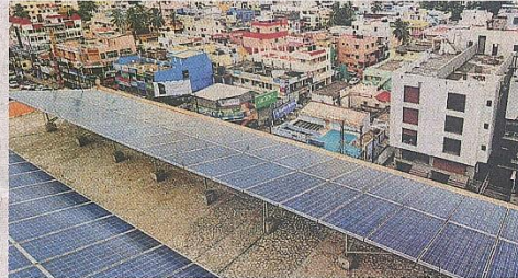
Low voltage: Roof size, right of use and costs are all issues in the residential sector, says Tata Power Solar's Khanna.
