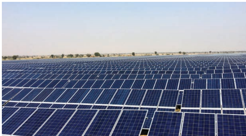
Large-scale solar projects accounted for 1,982 MW in the third quarter.
